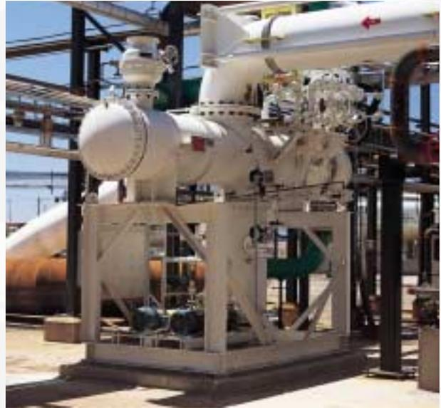
Mechanical drive turbine exhaust condenser at a U.S., West Coast chemical company.
