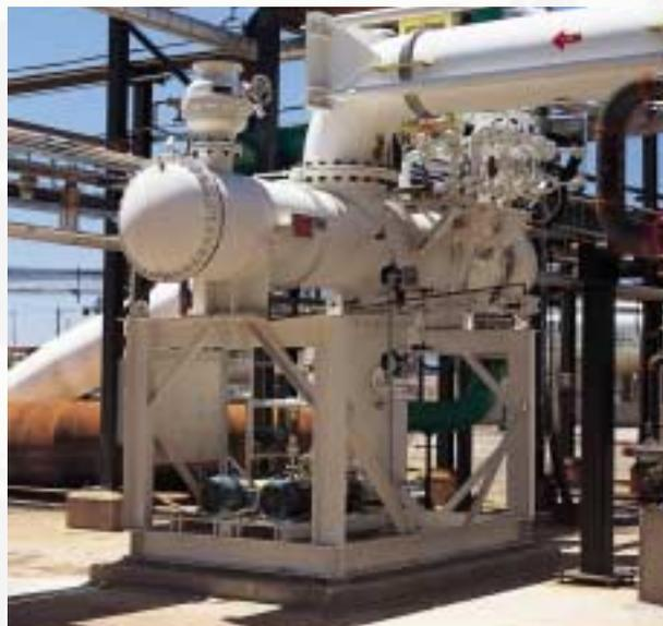
Mechanical drive turbine exhaust condenser at a U.S., West Coast chemical company.
