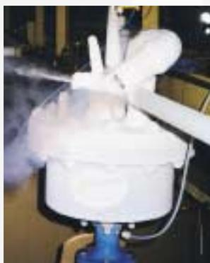
A cryogenically cooled vent condenser at a chemical storage facility that reclaims 98 percent of VOC vapors as condensate.
