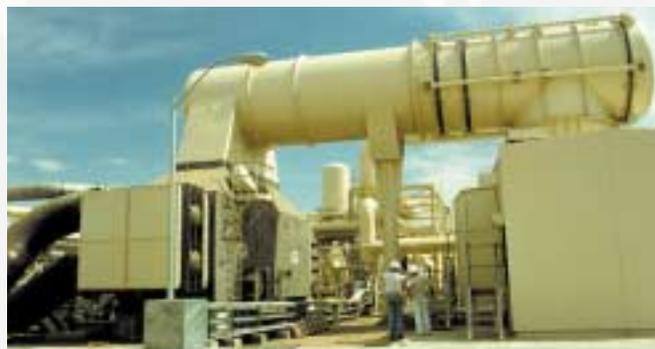
A large stainless steel condenser for a geothermal power plant on the U.S., West Coast
